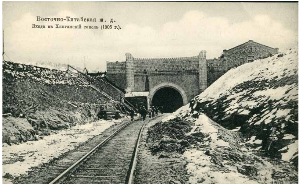
Fig. 7 The main Hingan Tunnel. One of eight such tunnels driven the mountainous terrain of the Hingan Range between Manchuli and Tsitsika during construction of the Chinese Eastern Railway.
