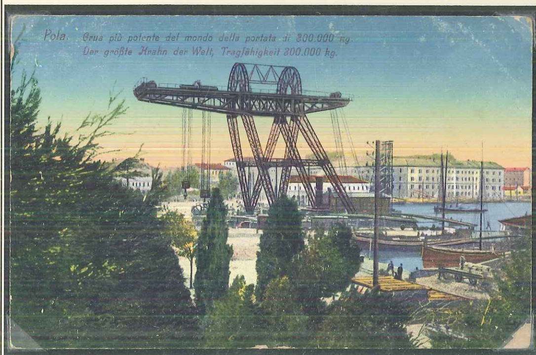
At that time. The largest crane in the world, lifting capacity 300,000kg
