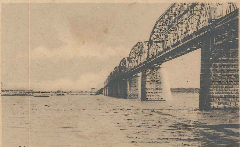
Harbin Viaduct on river Sungary
