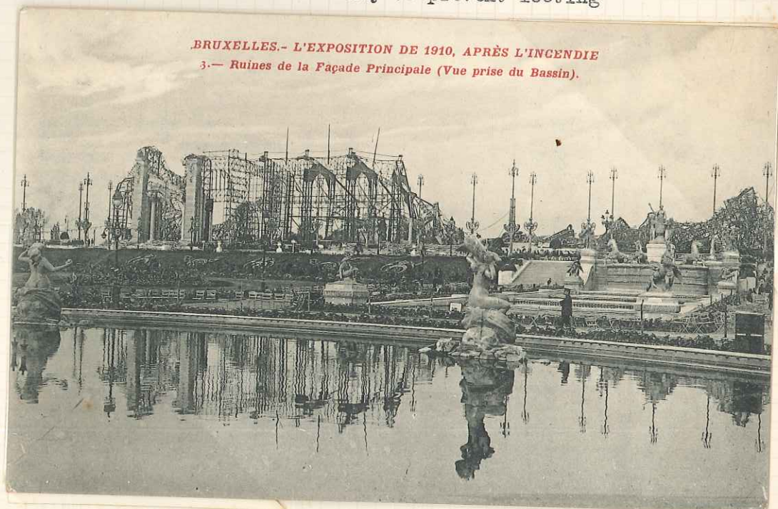
Ruins of the main Entrance and Facade
