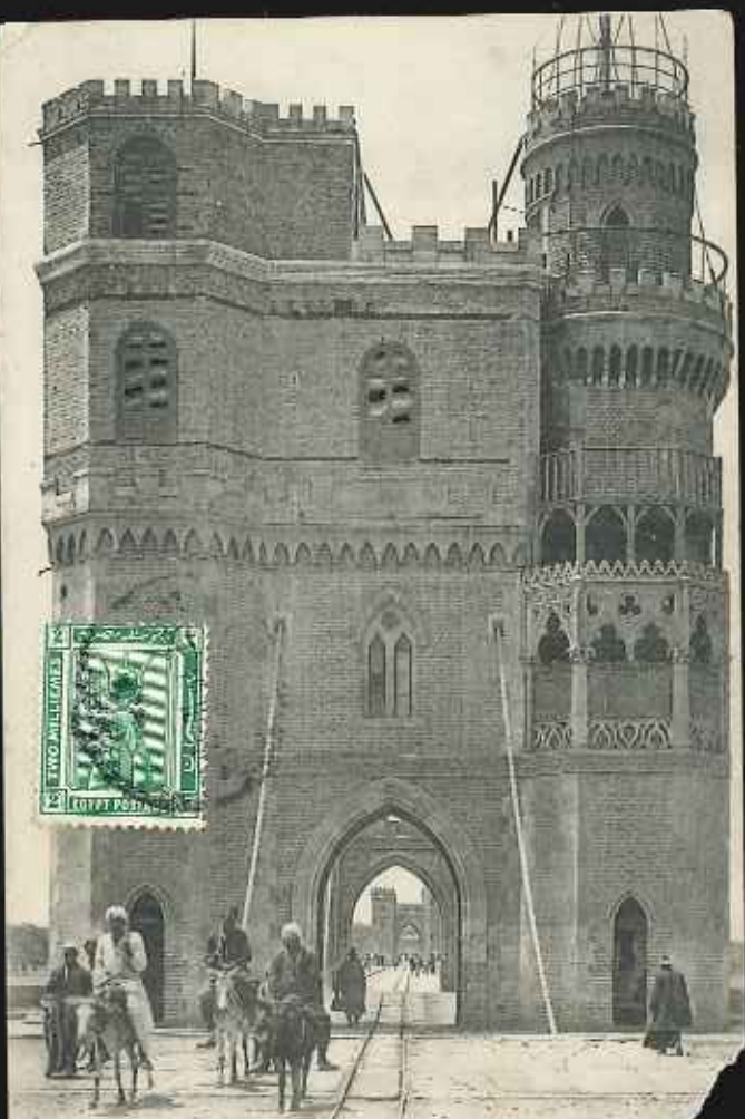
35 EGYPT. — Entrance to Great Delta Barrage — L.L.
